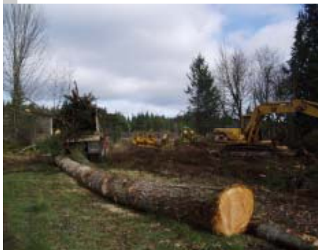
Road Clearing Project
